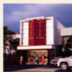
Poothole Branch (Car Parking Available)
